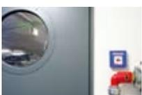
**5.** Due to the increasing formation of smoke, the fire alarm system automatically locks the fire door in the affected area.
