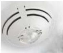
**2.** The fire detector detects the formation of smoke and transmits the information to the fire alarm control panel.
