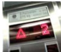
**6.** The fire alarm control panel takes over the elevator control and prevents the elevators from stopping in the affected areas and/or moves the elevator to a pre-defined end position.
